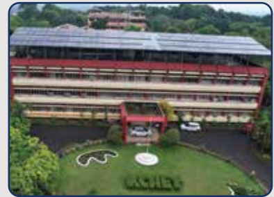
100kWp Solar Power plant at Kelappaji College of Agricultural Engineering & Food Technology, Malappuram
